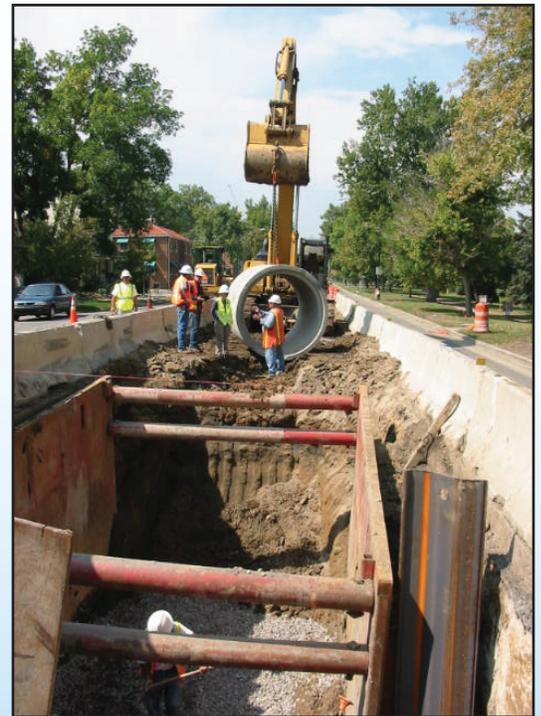
*Installation of 72-inch storm sewer in 17<sup>th</sup> Avenue*
