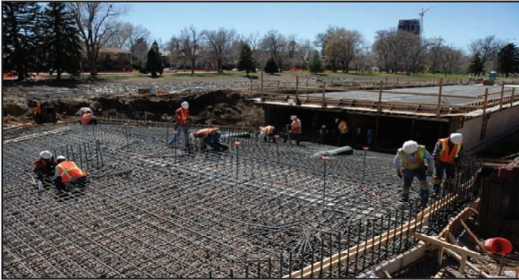
*Box culvert and construction of weir structure to control lake level and stormwater flow into the lake.*
