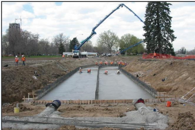
*Construction of lake Inflow Conduit - base slab of double 16'x 7' box culverts*
