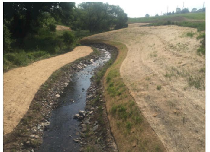
**Post-Construction Void-Filled Riprap on Weir Gulch.**
