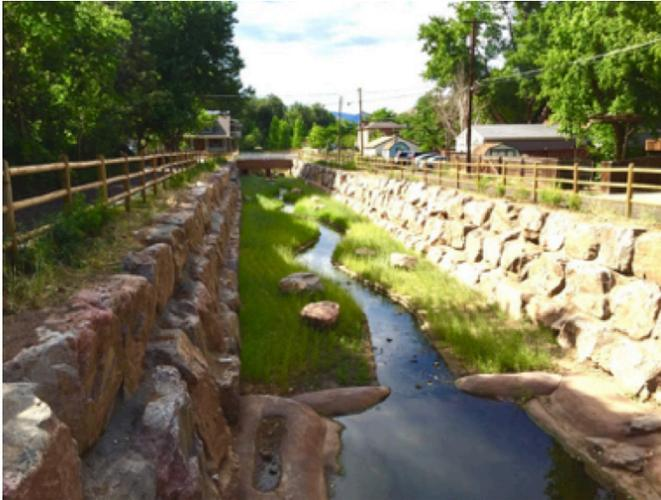
**Alleyway Boulder Wall Channel on West Fork of Kenney's Run - Envirolok® bags on bottom**
