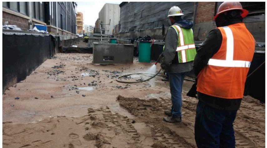
**A crew at Industry washes filter media into the structural base of this permeable pavement section. In the distance a second section will be constructed without filter media. Both sections will be monitored for water quality.**
