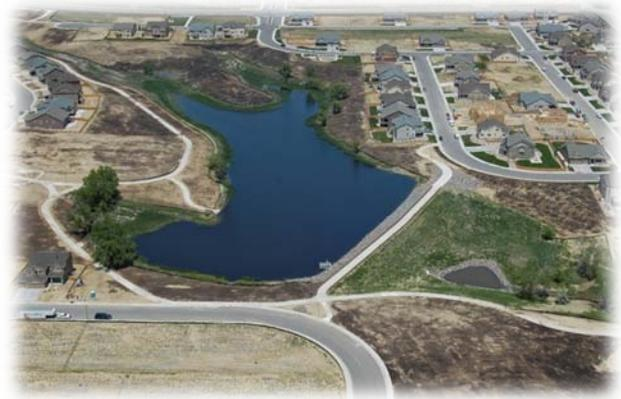
**Marshall Lake Dam, flood control was provided above the permanent water surface as a result of dam rehabilitation under the supervision of State Engineer's Office. Horizon Tributary to Brantner Gulch was stabilized throughout this development. 136<sup>th</sup> Avenue is visible in the background.**
