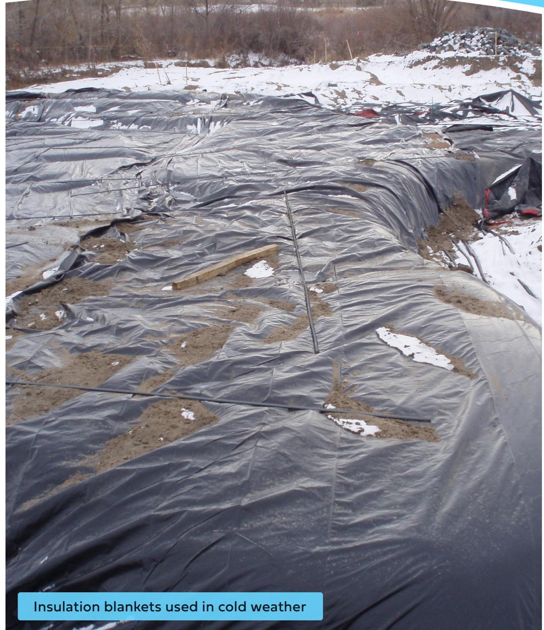
Insulation blankets used in cold weather
