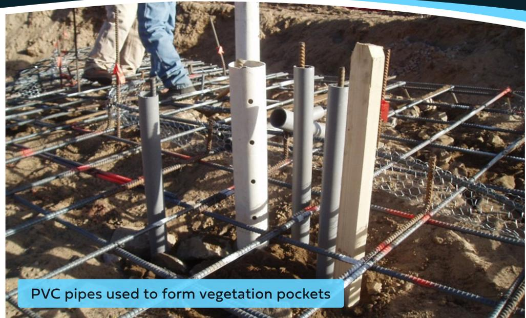
PVC pipes used to form vegetation pockets
