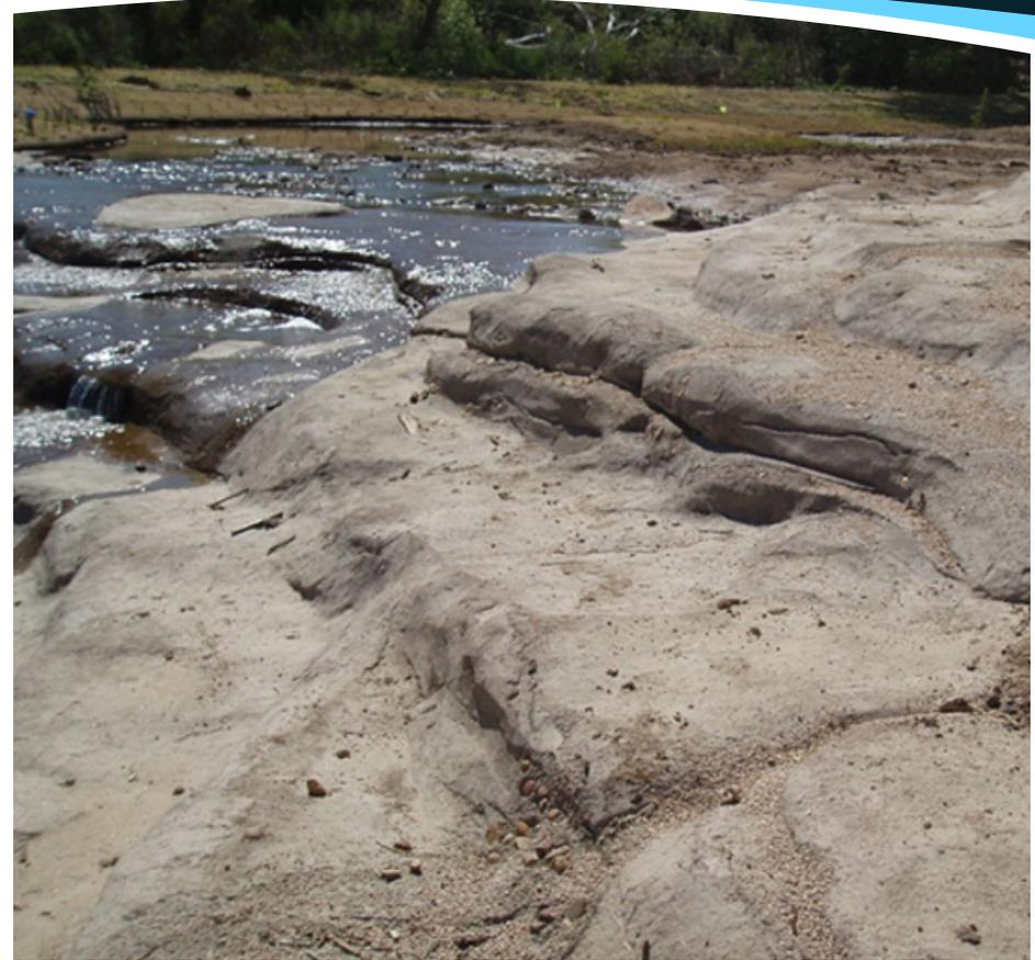
Subtle carving and shaping can often produce the desired finish. Notice the single horizontal carving through just one of the steps. Horizontal carvings on all the steps could look excessive and distract from the overall aesthetics.
