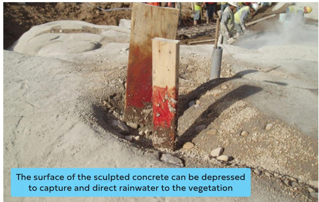
The surface of the sculpted concrete can be depressed to capture and direct rainwater to the vegetation
